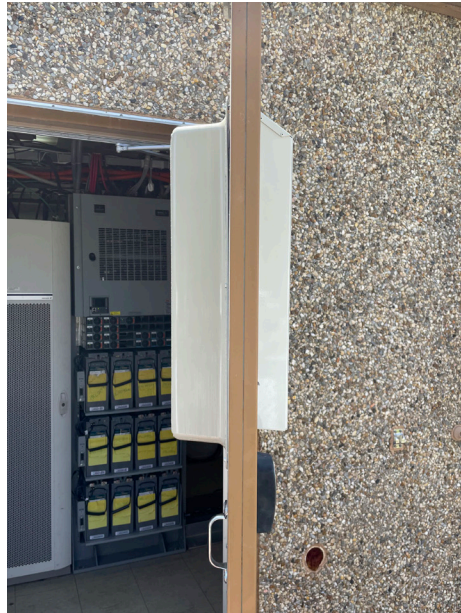
Left – exhaust cover, slim design; Right – exhaust damper
